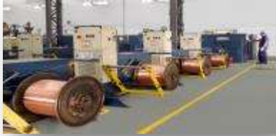
PVC Cable Factory
